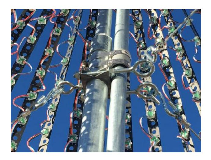
This guy wire mount design works perfectly with the ASAP Pole and could easily be adapted for other Mega Trees. It does not interfere with operation of the push pole or winch and allows for guy wires to be attached directly to the main pole.
